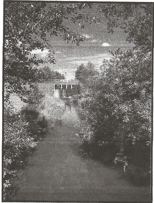
Luther Dam; West side of Millpond
